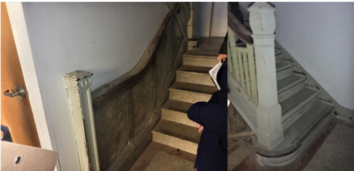
Figure 23: Existing stair of 120 Oxford Street
