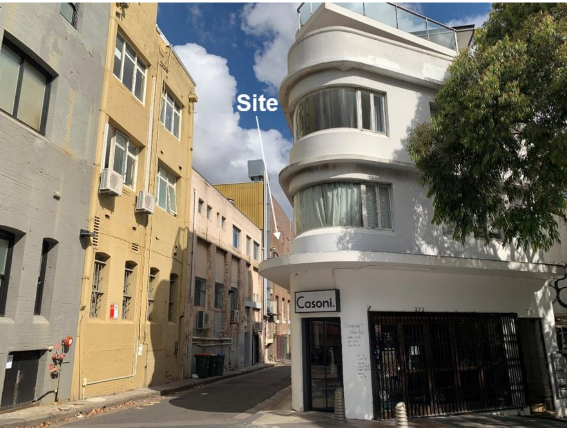
Figure 6: Foley Street as viewed from Taylor Square
