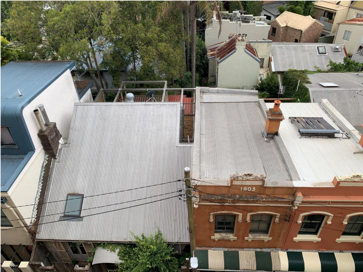
Figure 9: View from existing roof level to residential terraces on Foley Street
