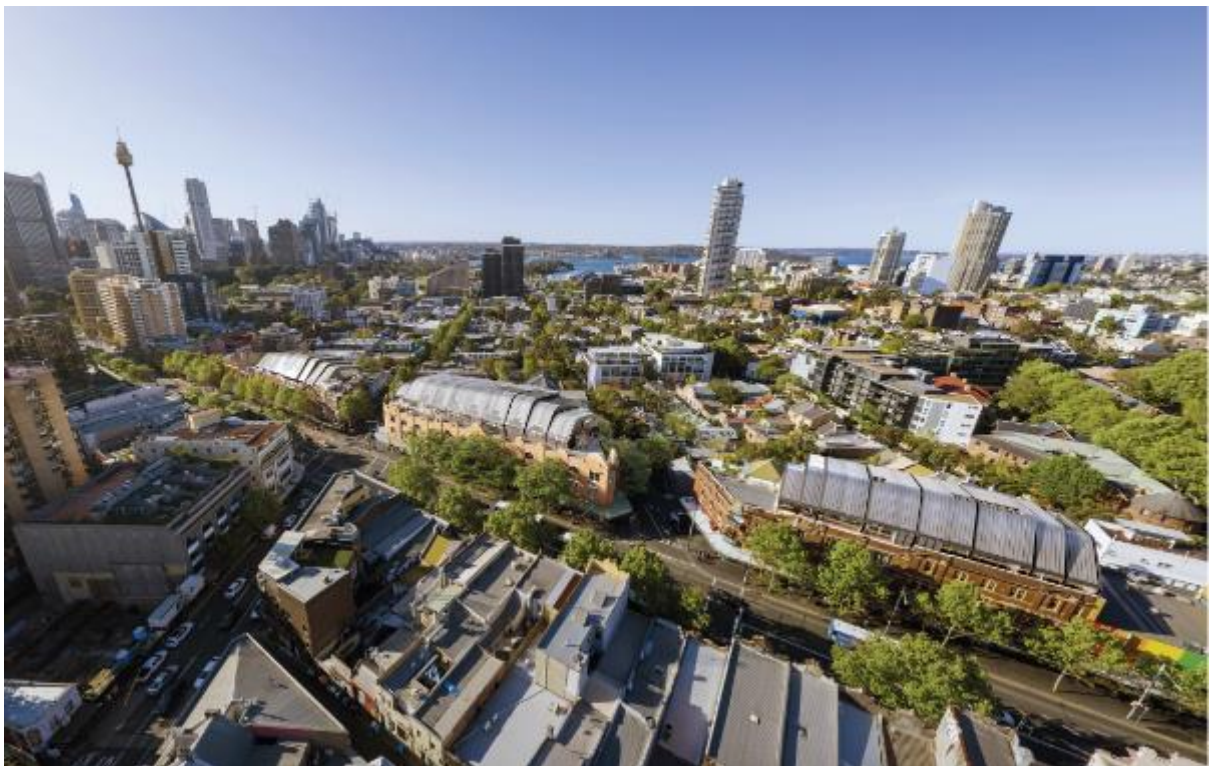
Figure 13: An aerial view of Group 1, Group 2 and Group 3 viewed from the south-west (Note: Groups 1 and 2 are not the subject of this report)
