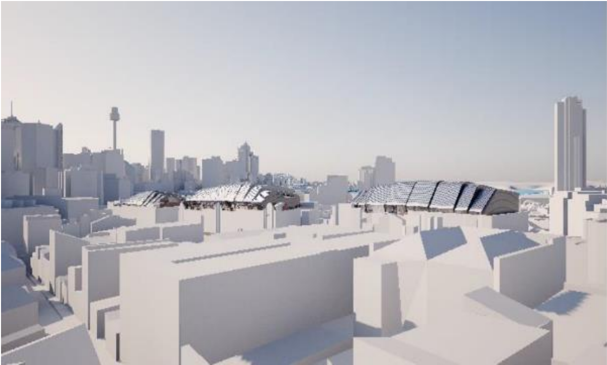
Figure 31: Modelling from applicant's view loss study, as viewed from Level 5 of 200 Campbell Street
