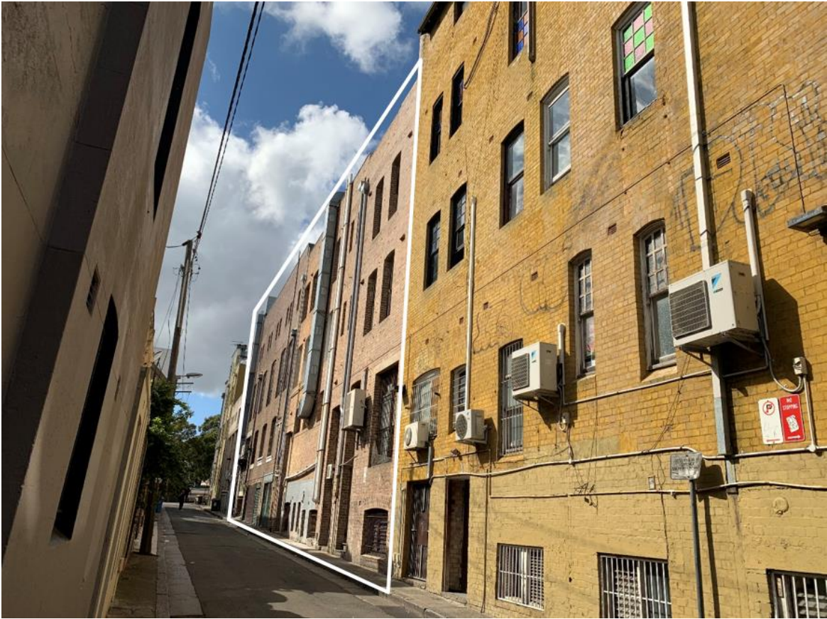
Figure 3: The site viewed from Foley Street
